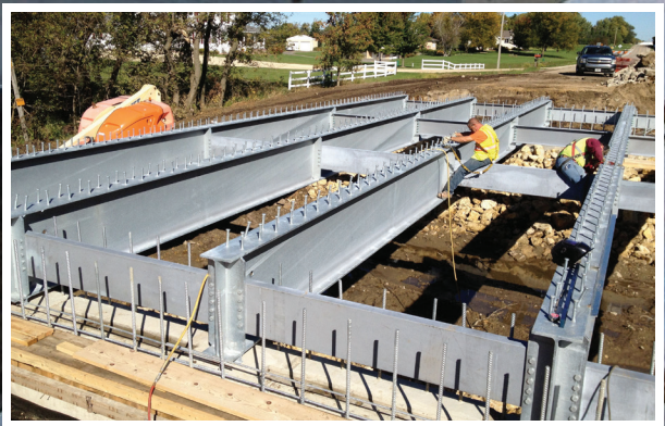
Construction of Bridge with Galvanized Steel Beams – Buchanan County, Iowa; Photo credit: American Galvanizers Association
